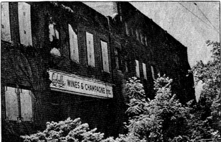
The old abandoned LaSalle winery on Grand River will soon become the home for several wholesale firms and a theme restaurant as its new owner finalized the real estate transaction last week and made plans for remodeling the 96-year-old structure. (Staff photo)
